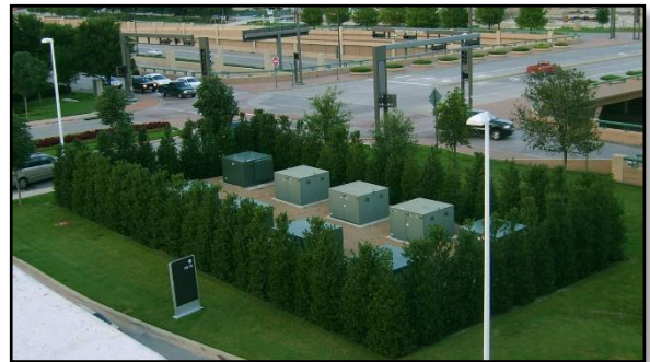
Figure 18: Example of Screened Ground-Mounted Utility Equipment
