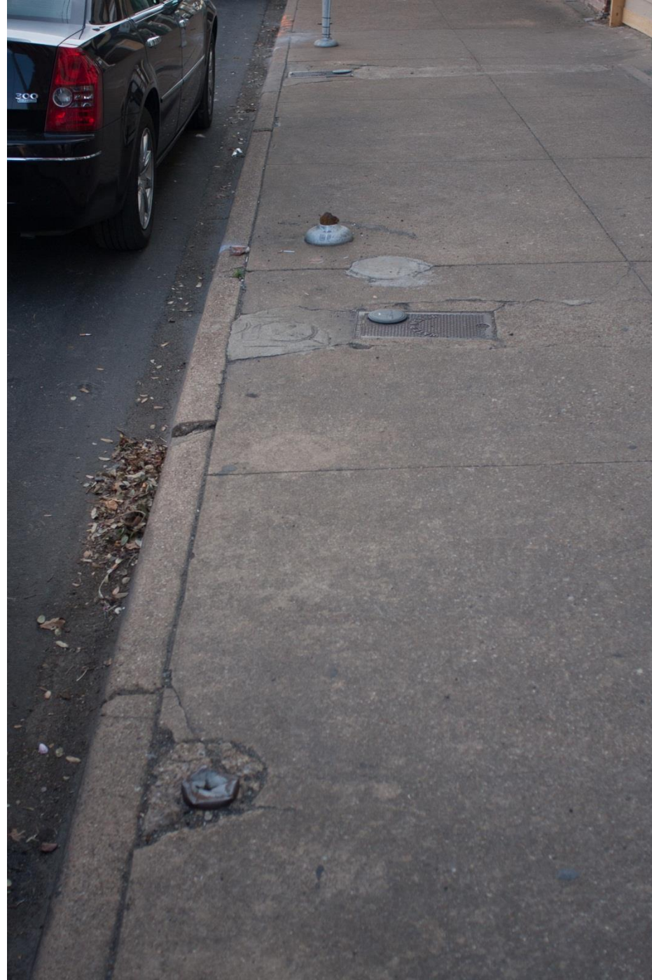
Throughout the area, utility meters, grates, stumps where parking meters formerly stood, and other surface obstacles present potential accessibility and aesthetic issues. Location: non-specific.
