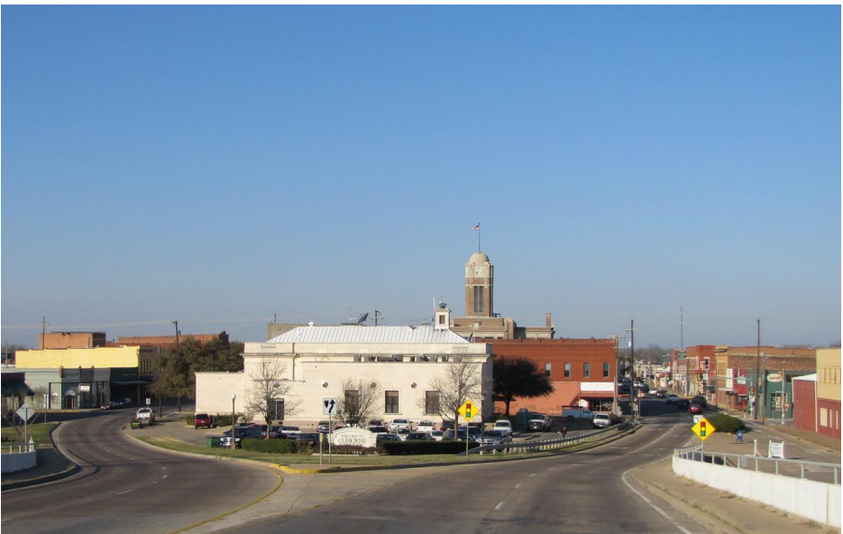
View from the overpass along SH67
