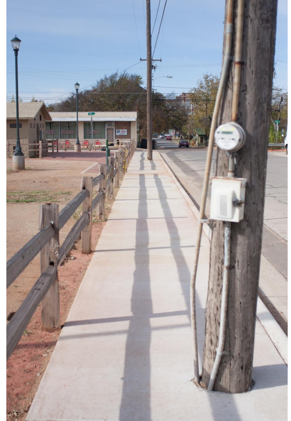
The location of utility poles in this new sidewalk impacts its aesthetic character and makes it more challenging for people in wheel chairs or couples walking abreast. Location: Harrell Street along Market Square.
