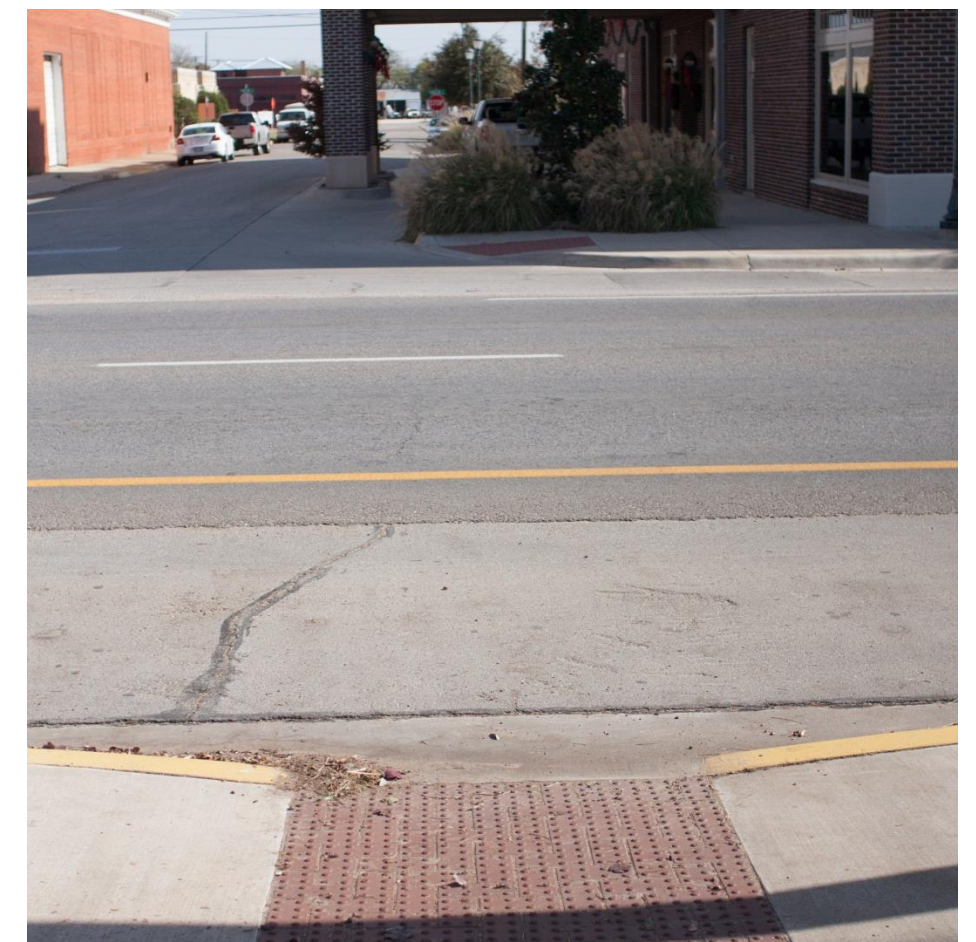
New sidewalks were built around the Wright Place building. These represent the most-accessible sidewalks in the best condition. However, there are instances where marked crosswalks and no-parking zones are missing, rendering curb ramps ineffective. Location: Caddo Street at James Street
